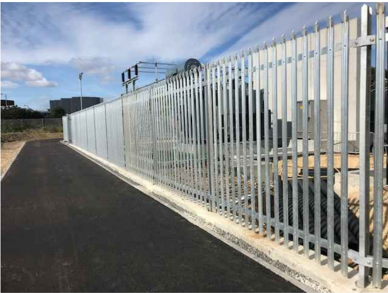
TYPICAL FENCE INSTALLATION
